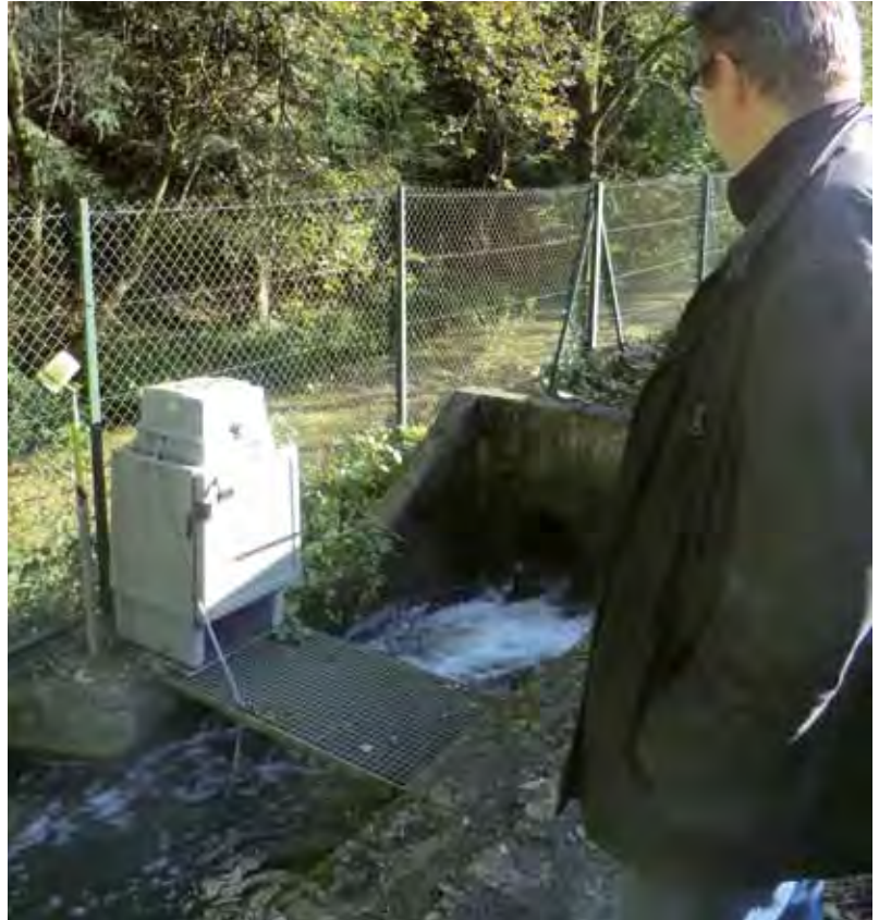
Monitoring next to a sewage facility in the Mamer river basin
